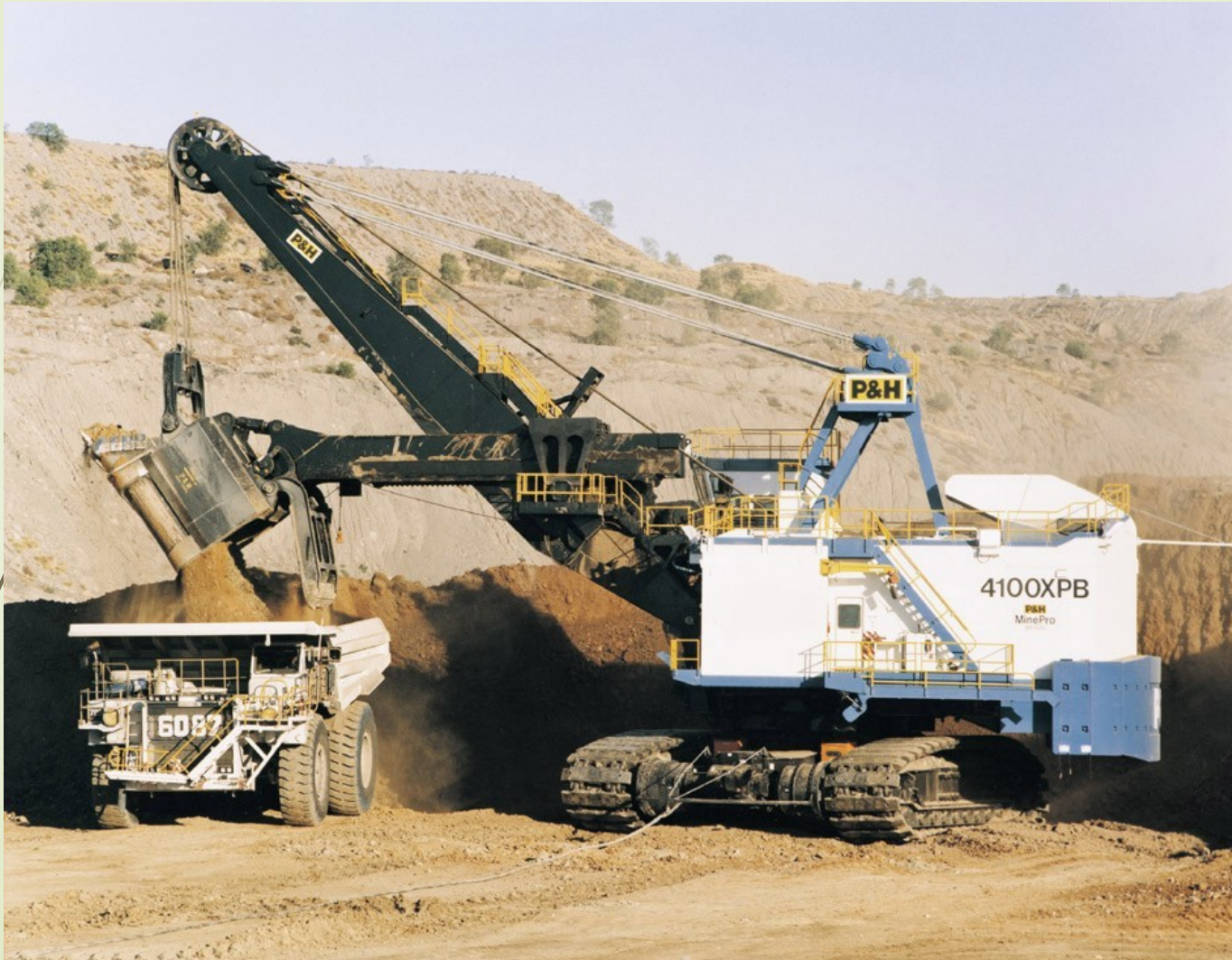
2500kVA 11000-6600/600-600V Cast Resin Transformer AN IP43 on a Mine Shovel
